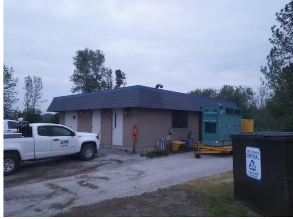
IMAGE 7 GRAVEL DRIVEWAY AND CONCRETE BUILDING
