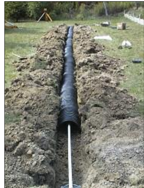
Single line shallow buried trench.
