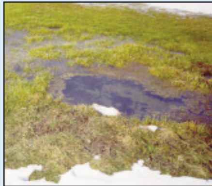
Effluent pond on top of the leaching bed.
